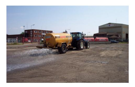
Dustbuster 1 is a dust wetting additive consisting of a blend of special surfactants which inrease the ability of water to wet and suppress road dust.
